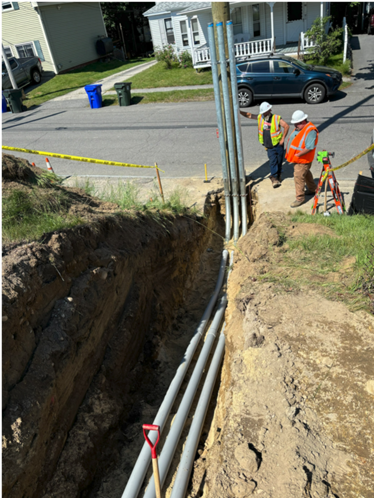
U/G Electrical work from CT cabinet to future pole-mounted transformers
