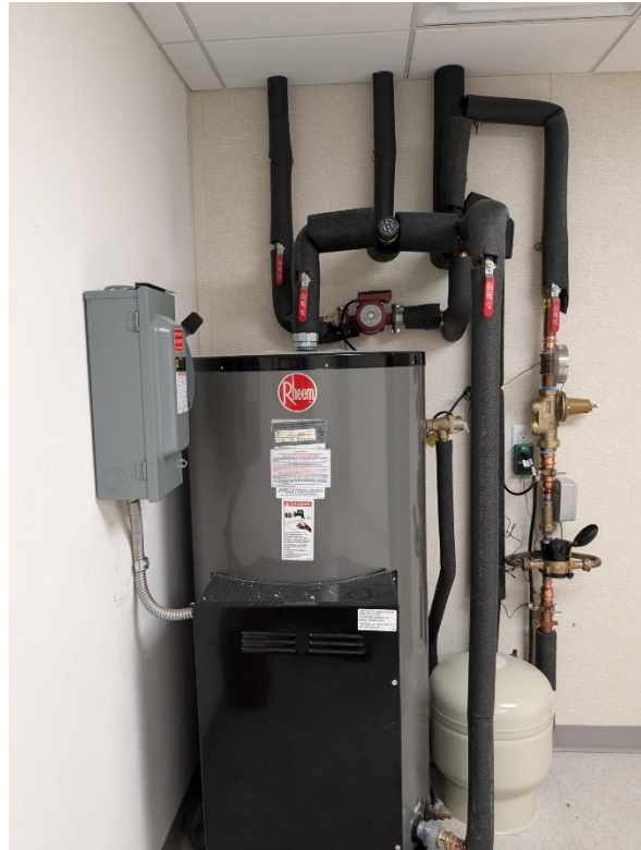
Water heater installed and expansion tank installation
