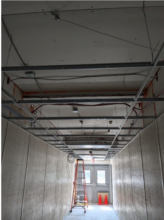
Ceiling grid framing ongoing
