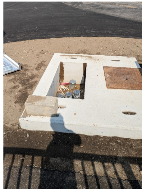
Transformer pad ready to receive the pad mounted transformer
